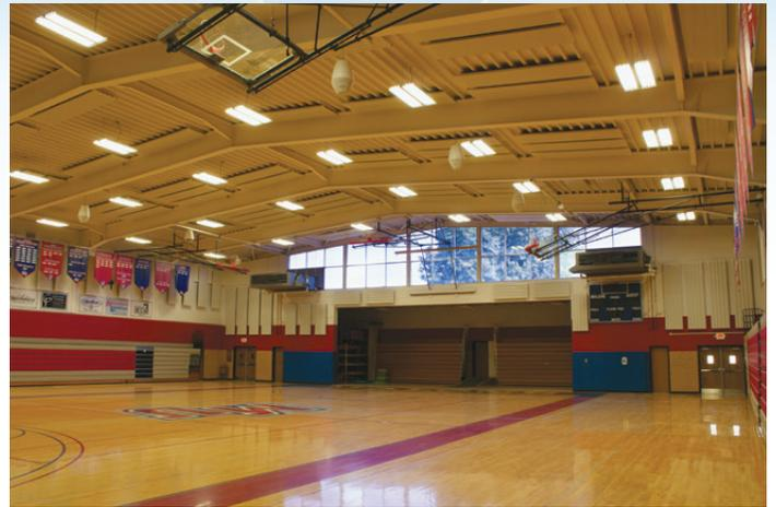
*absorption at the most critical frequency to suit Malone's acoustic requirements. Plus, Eckel EFPs offer superior durability to withstand impacts from basketballs, soccer balls and the like."*
